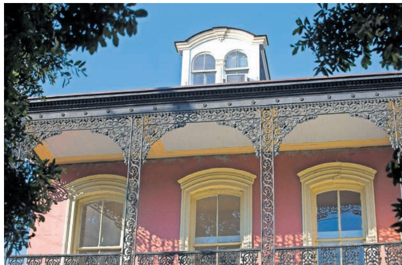
Above: Italianate segment arches frame the windows at 1235-37 St. Andrew St.
