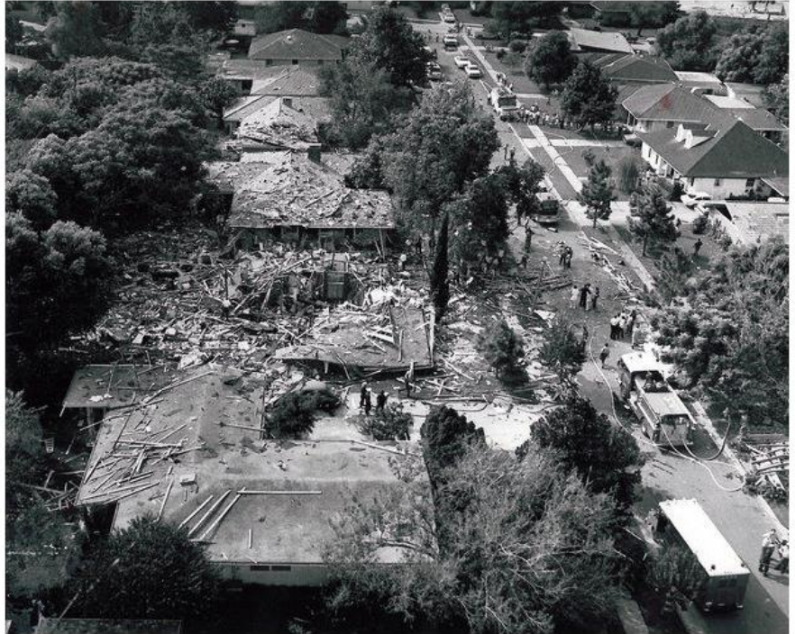
An explosion in the early hours of Sept. 1, 1975 ripped apart this Metairie residence in the Bissonet Plaza area. The blast, which injured five members of the Stephen M. Little family and six of their neighbors, was believed caused by a gas leak. But an underlying cause was soil subsidence. An eyewitness described the 8:45 a.m. explosion as looking “like a bomb going off.” Eight other houses in the immediate area received structural damage. (G. E. Arnold, NOLA.com | The Times-Picayune archive)
