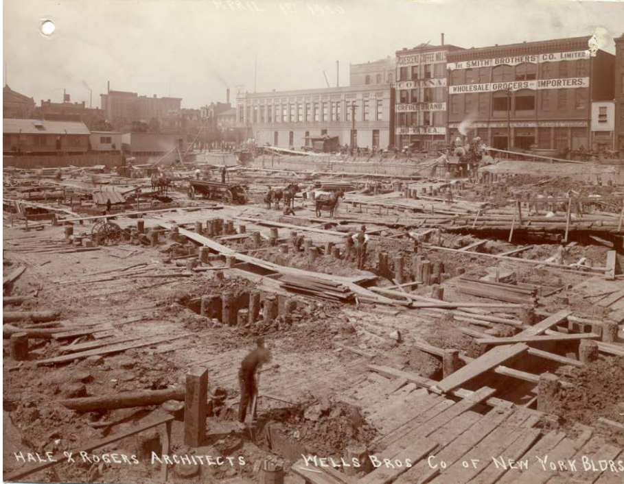
1910 site preparation at 600 Camp; photo courtesy Court of Appeals.
