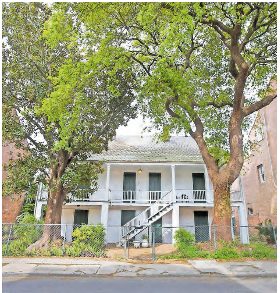
The Ossorno House, at 913 Gov. Nicholls St., is an example of 18th-century Creole architecture. It was moved from Bayou St. John to its French Quarter location in 1784. Chris Granger / staff archive
