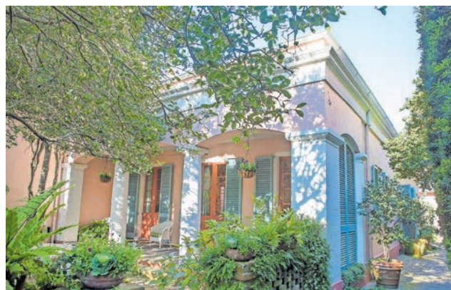
The earliest known surviving structure in New Orleans with prominent Greek traits is the Thierry House (1814) at 721 Gov. Nicholls St.
