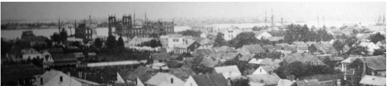
Ruins of Touro's Alms House appear in the distant left of this 1867 detail taken from Holy Angels Convent in present-day Bywater. Courtesy Tulane Southeastern Architectural Archive.
