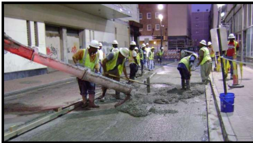
Top: Repaving on Toulouse Street at Bourbon in 2012 uncovered old paving stones and the curve of a streetcar track bed (photo by Richard Campanella). Middle: Comparison of patchy asphalt composite surface at left and new concrete surface at right, on lower Julia Street (photo courtesy City of New Orleans). Bottom: Workers pouring new concrete surface on Iberville Street in 2016 (photo courtesy City of New Orleans).
