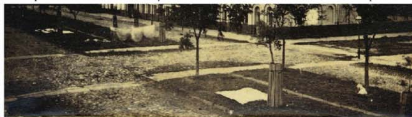
Streetscape by the Parish Prison in the Faubourg Tremé, circa 1864. Note the paving blocks used for the crosswalks, designed to give pedestrians a slightly smoother stroll than smaller rounded paving stones. Detail of photograph from Marshall Durham Collection, Louisiana State Museum, used with permission.
