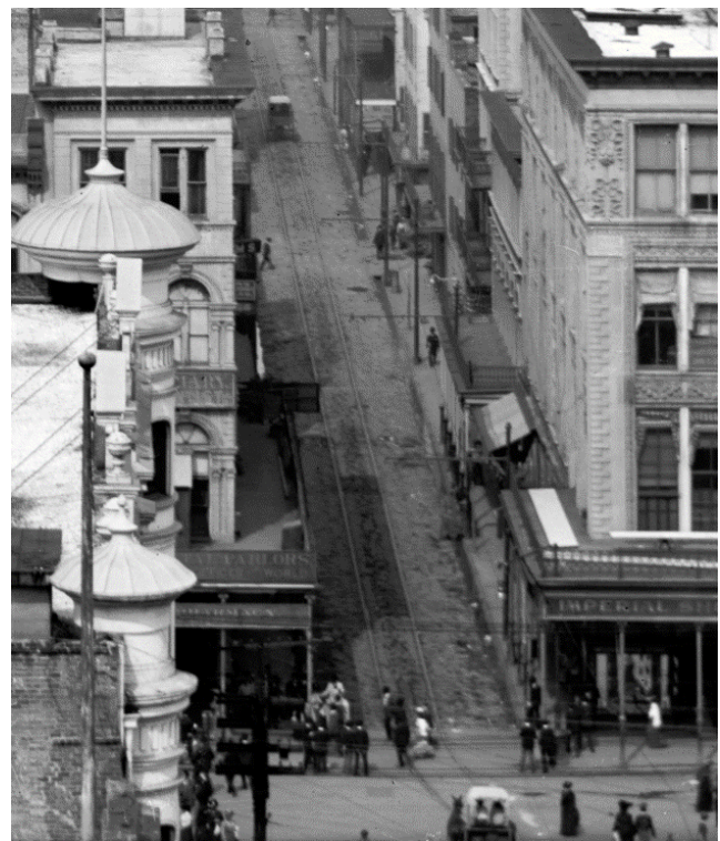
This c1900 rooftop view up 100 Bourbon shows paving stones and streetcar rails for the line that later served Desire Street. Photo courtesy Library of Congress.
