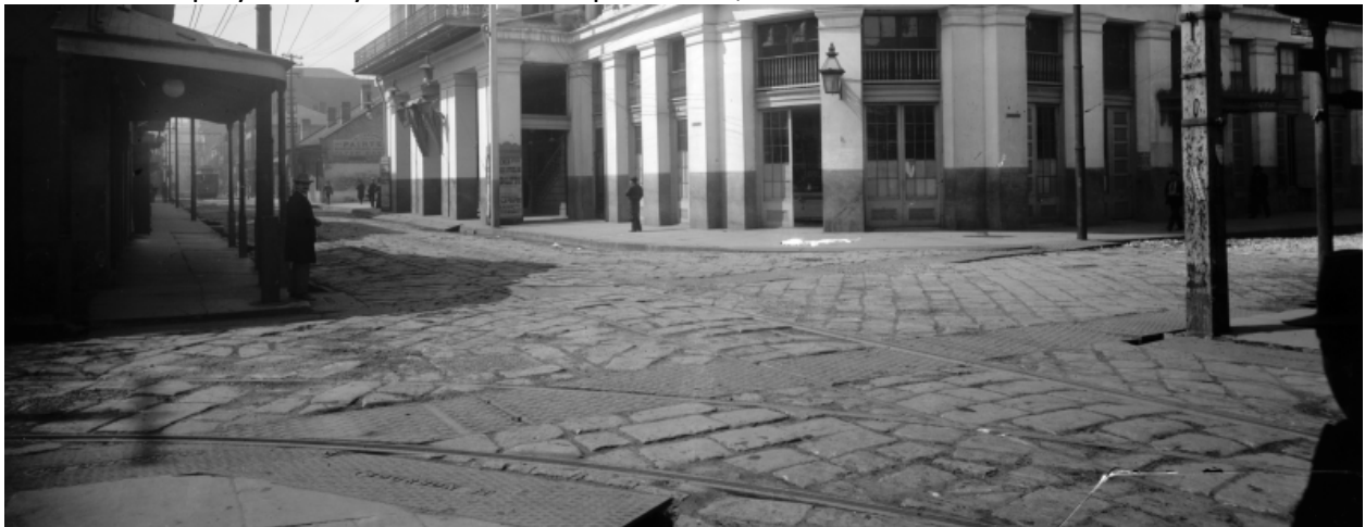
Paving stones and steel walkways set among streetcar rails on Bourbon Street at Toulouse by the Old French Opera House, c1900. Photo courtesy Library of Congress.
