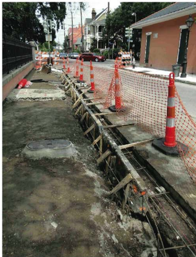
New sidewalks installed along Royal and Esplanade in August 2012. Note the reutilization of old granite paving blocks to form the curb.
