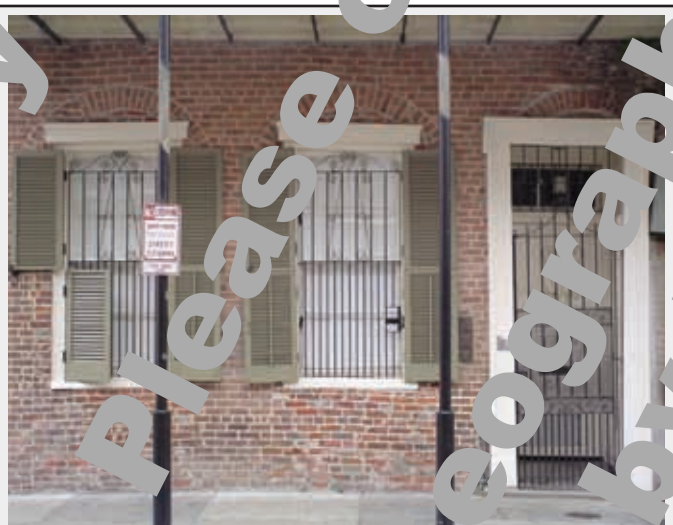
Bourbon Street example of arched openings, typical of pre-1830s Creole style, renovated into arched openings and a “keyhole” entrance, typical of circa-1840s Greek Revival style. Photograph by author, 2004.
