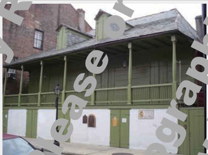
“Mada John’s Legacy” (632 Dumaine). Built immediately after the 1804 fire, exhibits classic traits of “first-generation” Creole architecture: an oversized double-pitched hip roof, center chimney, colonnades supporting airy gallery, outdoor staircases and no internal hallways. All raised high on brick piers. One can visualize colonial New Orleans by picturing scores of similar structures, in various sizes, setbacks, and orientations. Photograph by author, 2004.
