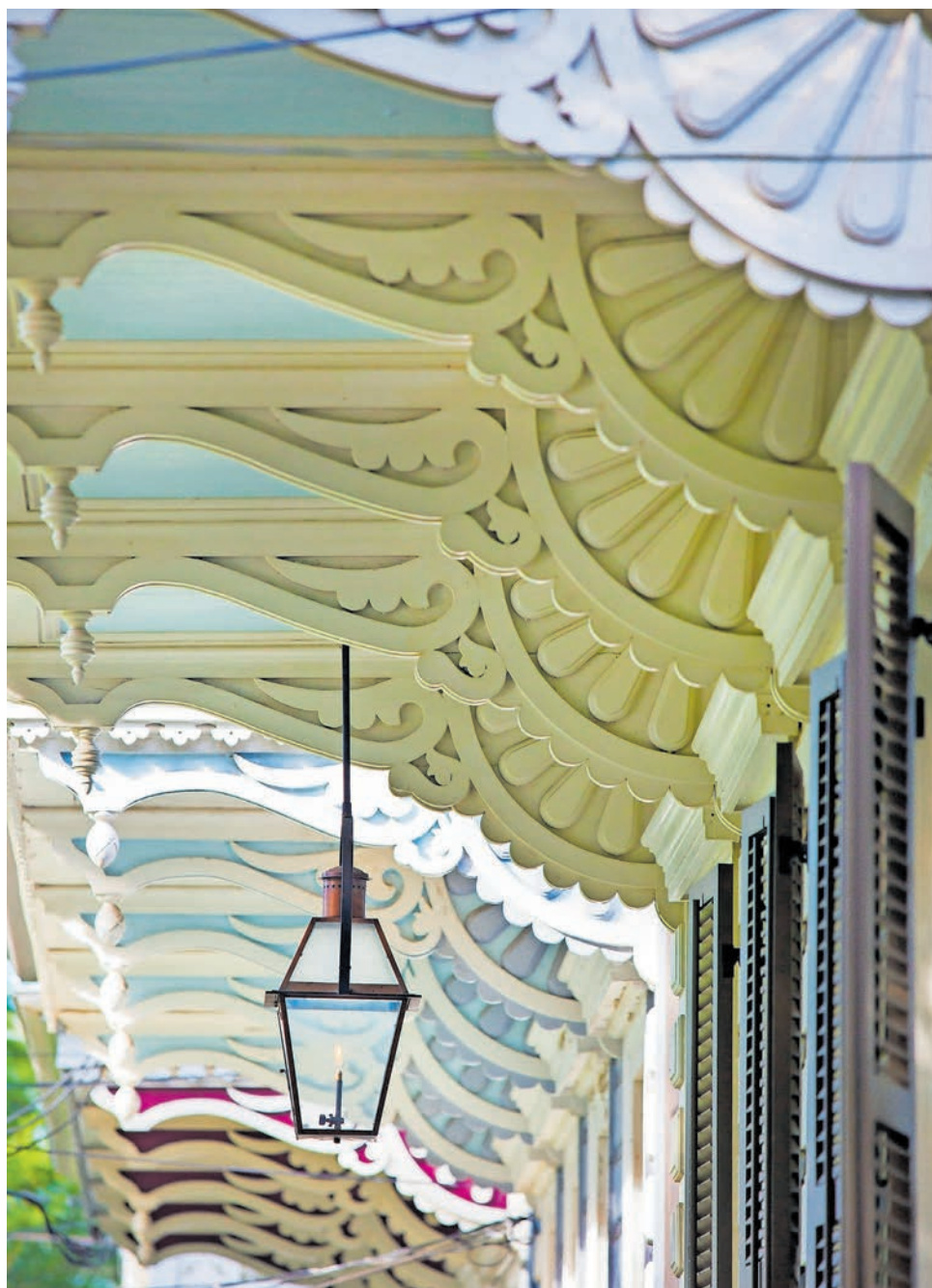
By the end of the 19th century, late Victorian architectural styles, such as Eastlake and Queen Anne, absorbed Italianate's penchant for elaborate detailing, and builders milled brackets and quoins en masse to spruce up shotgun houses. Chris Granger / cgranger@nola.com
