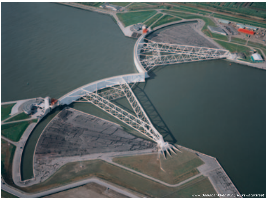
Maeslant Storm Surge Barrier in the Rhine-Meuse delta
