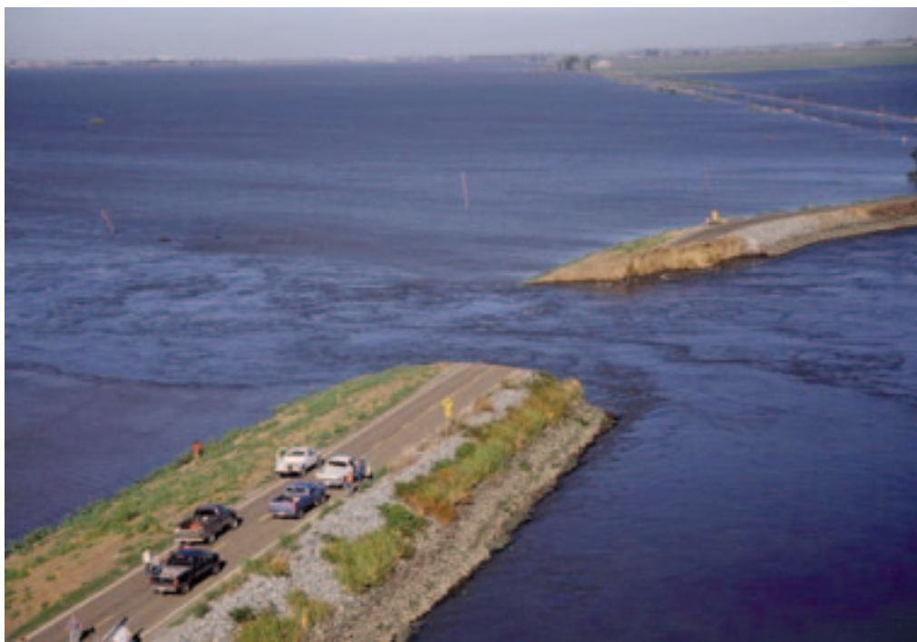
Levee failure in California Bay-Delta
