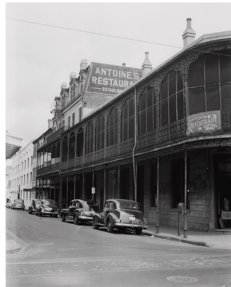
Antoine's Restaurant previously had an enclosed gallery, as shown here in this photo from the 1940s. Image courtesy of The Historic New Orleans Collection.
