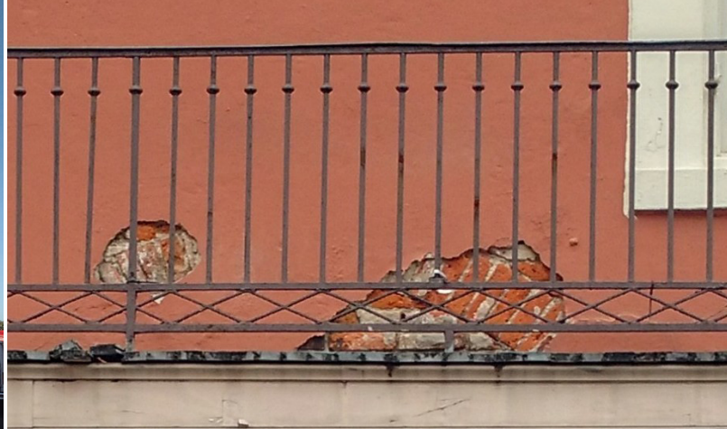
LEFT: Spanish-style brick arch revealed behind stucco of 601 Chartres St. RIGHT: Exposed brick under stucco at 601 Chartres St. Photos by Richard Campanella.
