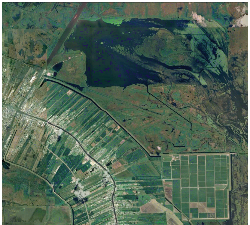
This recent satellite image shows how Delta Farms has filled with water, the consequence of its levee having failed, and its terrain having subsided below sea level. Clovelly Farms, at lower right, which remains in operation, sits at 4.5 to 6.5 feet below sea level. RICHARD CAMPANELLA
