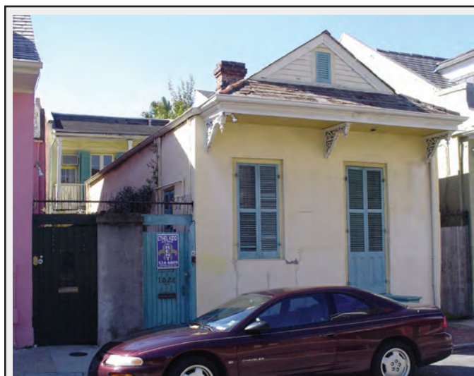
The Vieux Carré Survey described 1028 St. Philip as follows: "Originally this c. 1839 single, long brick cottage was approximately 3' lower in height [than] it is today. A massive c. 1880 renovation, which included a roof change and a possible raising in height transformed the early cottage into a late 19th c. single shotgun." Thus there are two construction dates (1839 and 1880), two styles (arguably Creole and Victorian), and two structure types (cottage and shotgun) manifest in a single building. Note the quarters in the rear, a rarity for shotguns. Photograph by author, 2004.
