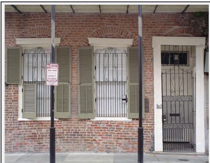
Bourbon Street example of arched openings, typical of pre-1830s Creole style, renovated into squared openings and a “keyhole” entrance, typical of circa-1840s Greek Revival style. Photograph by author, 2004.
