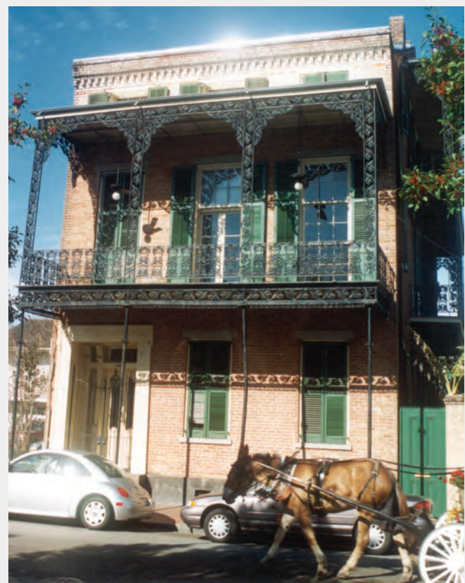
This townhouse at 1025 St. Louis Street is one of the finest examples of the Greek Revival style in the Quarter. Built in 1840-1842 for two free men of color, the 7,600-square-foot mansion's Greek key doorway, side hall, squared openings, heavy lintels, attic windows, and dentils are classic traits of this antebellum style. Photo by author, 2002.
