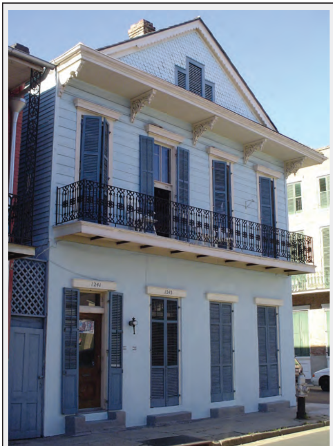
Cottages from the colonial and antebellum eras were often razed for postbellum frame and shotgun houses. In other cases, the aged units were simply appended. 1201 Bourbon is a good example: the lower floor was once a circa-1840 Creole corner cottage with Greek Revival details, to which Victorian-style upper floors were added in the late 1800s. Photograph by author, 2004.
