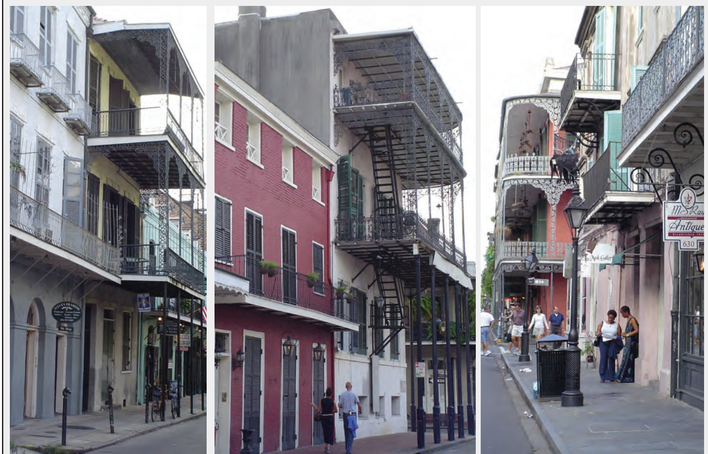
Balconies span half the width of the banquette (sidewalk) and are usually supported by cantilevers; earlier examples in the French Quarter incorporate wrought iron and tend to be simple and strong. Galleries cover the entire banquette, are supported by cast-iron columns and lace, and form semi-enclosed, semi-private space. They became popular around 1850, permanently transforming the New Orleans cityscape. In these photographs, balconies appear in the foreground, and galleries in the rear. Photographs by author, 2004.
