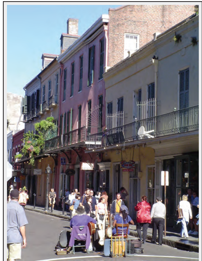
The 600 block of Royal Street possesses fine examples of Spanish-influenced "second-generation" Creole architecture. At right is the Ducros-Ducatel House and its additions (1805-1825), exhibiting a stucco entablature with moldings, steep hip roof (not visible here), narrow balcony, arched openings on the ground floor (later squared), and a dependency with wooden railings and colonnades. Next door is 610-614 Royal, a pink three-story townhouse in the "high Creole" style of the 1830s, with a central porte cochère and unadorned double-hung windows topped with stucco-covered jack arches. The adjacent units at 616-624 Royal were built in the same era and style. Graceful, smooth simplicity uninterrupted by cluttering detail typifies these Creole styles. Photograph by author, 2004.
