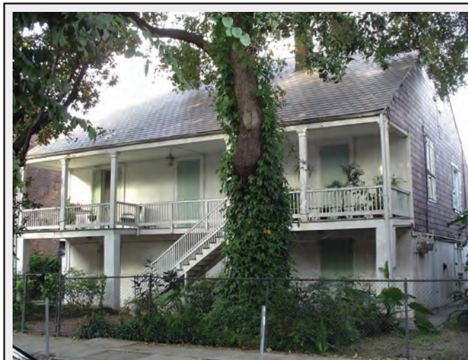
The oldest extant structure in the rear of the Quarter is the remarkable Ossorno House. A plantation house by design, origin, and function, it was apparently dismantled from Bayou St. John around 1781 and reassembled at present-day 913 Gov. Nicholls by 1784. Although its original West Indian-style hip roof had been remodeled to a gable by the 1830s, the house is still distinctly rural in appearance, orientation, and setback. It is an amazing exception to the French Quarter cityscape, like an old Dutch farmhouse in New York City or Spanish mission in Los Angeles. Photograph by author, 2004.
