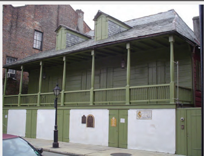
“Madame John’s Legacy” (632 Dumaine), built immediately after the 1788 fire, exhibits classic traits of “first-generation” Creole architecture: an oversized double-pitched hip roof, center chimney, colonnades supporting an airy gallery, outdoor staircases and no internal hallways, all raised high on brick piers. One can visualize colonial New Orleans by picturing scores of similar structures, in various sizes, setbacks, and orientations. Photograph by author, 2004.
