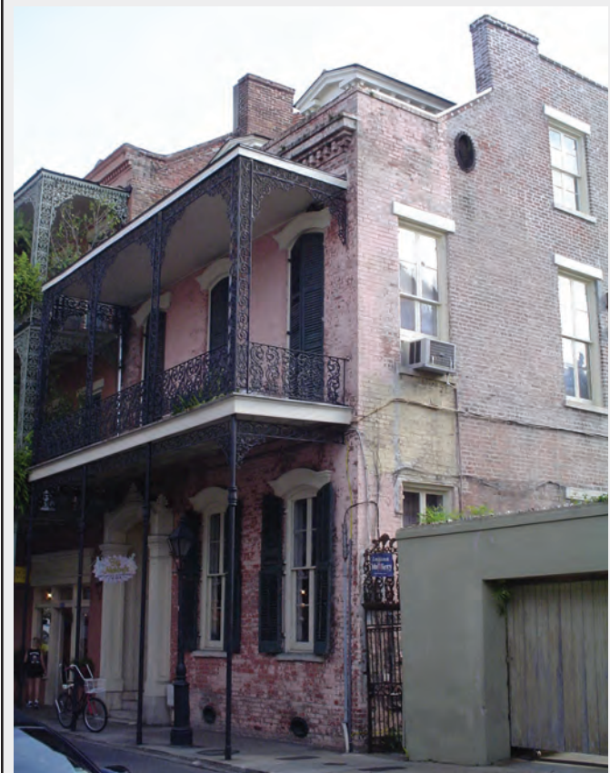
This late-1850s townhouse at 934 Royal illustrates the transition from Greek Revival to Italianate. The heavy lintels above the side windows are Greek Revival traits, while the decorative parapet and segmented arches on the façade are Italianate. Photograph by author, 2004.
