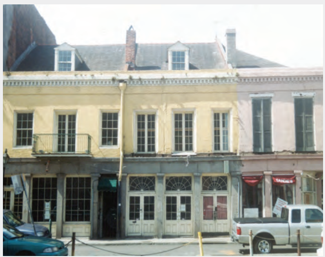
This row of “transitionals”—structures with both Creole and Greek Revival traits—at 335-341 Chartres dates from the 1830s, when political power shifted from Creoles to Anglos. Creole traits include the narrow balcony, jack arches above windows, and narrow passages between adjoining units; Greek Revival characteristics include the denticulated cornice, squared openings, and massive granite pillars. Photograph by author, 2002.
