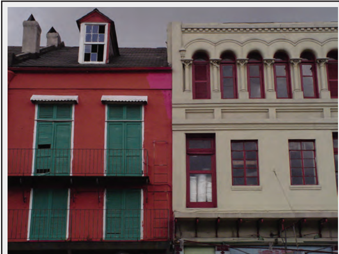
Contrasting nineteenth-century styles at 913-915 Decatur: at left is a circa-1830s Creole-style storehouse; at right is a Roman Revival-style façade dating from the 1890s. Photograph by author, 2002.
