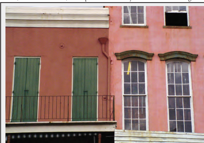
Another contrasting pair at 1027-1035 Decatur: at left is a Creole-style structure in a row of three built around 1829; at right is a Victorian Italianate commercial building built in 1883. Note the simple, clean lines of the earlier, indigenous style compared to the fancy traits of the late nineteenth-century imported style. Photograph by author, 2002.
