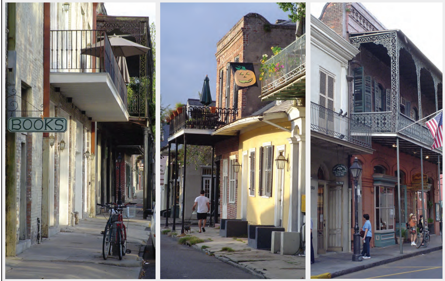
Balconies span half the width of the banquette (sidewalk) and are usually supported by cantilevers; earlier examples in the French Quarter incorporate wrought iron and tend to be simple and strong. Galleries cover the entire banquette, are supported by cast-iron columns and lace, and form semi-enclosed, semi-private space. They became popular around 1850, permanently transforming the New Orleans cityscape. In these photographs, balconies appear in the foreground, and galleries in the rear. Photographs by author, 2004.
